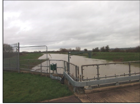
View from River Witham sluice gates looking north towards location of proposed bridge
